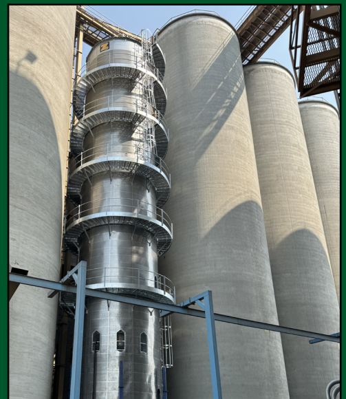
The new dryer being installed at the Bisbee terminal will double drying capacity from 5,000 bushels per hour to 10,000. If progress continues as it has, it should be ready for drying corn this fall.
